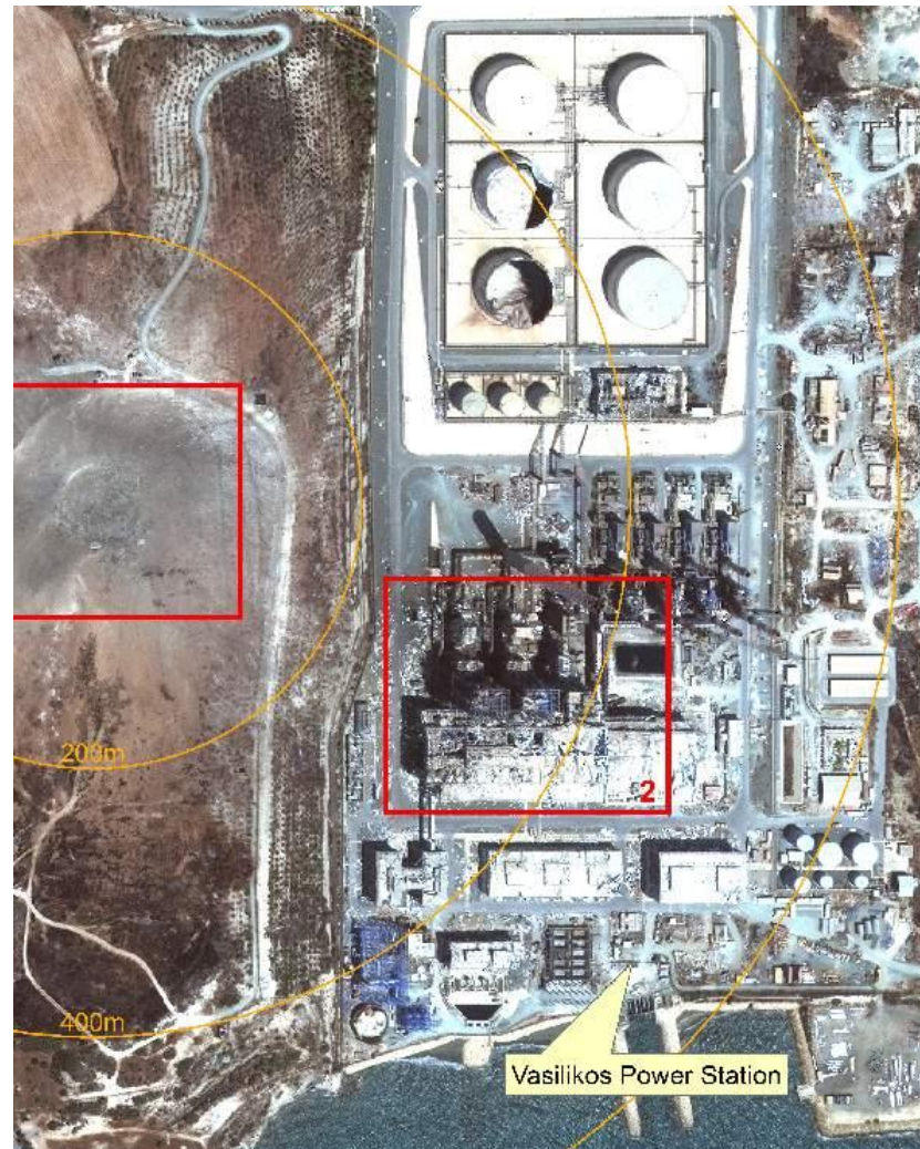
Figure 68 - Vasilikos Power Station incident
