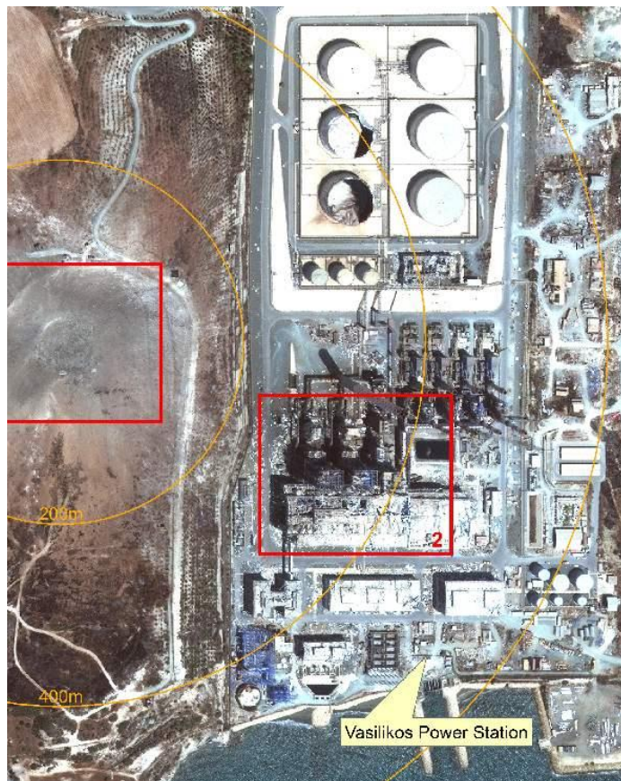
Figure 69 - Vasilikos Power Station incident
